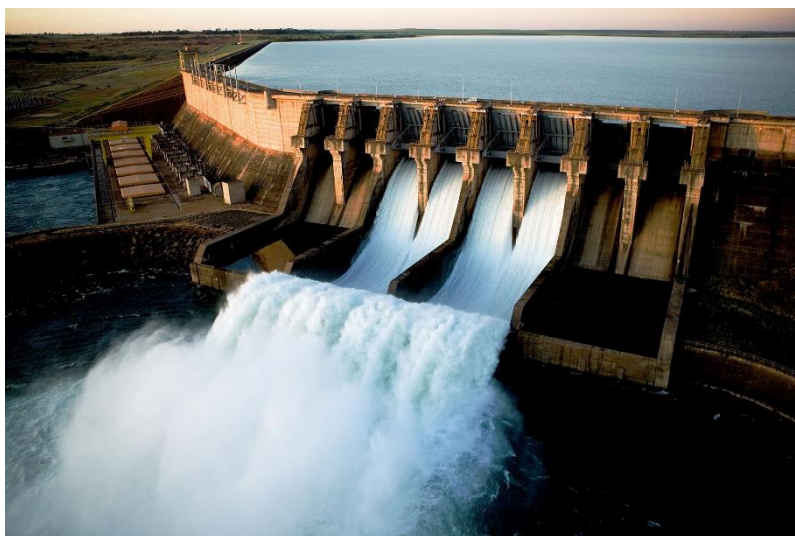
Figure 6 - Hydroelectric power station
